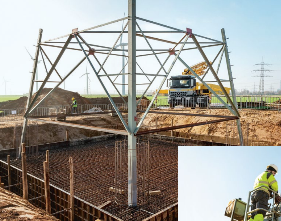
Milestone in the "Rheinschiene" grid expansion project: the first pylon foundation under construction.
