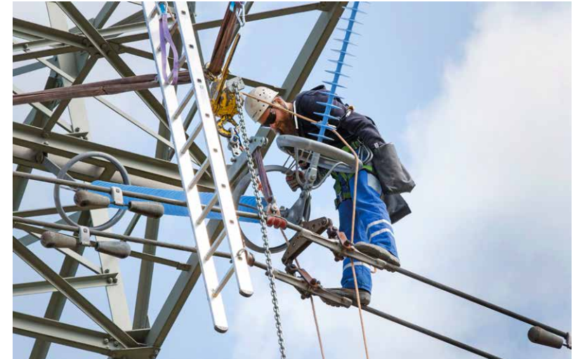
DC transmission systems such as Ultranet enable electricity to be transported particularly efficiently over longer distances.
