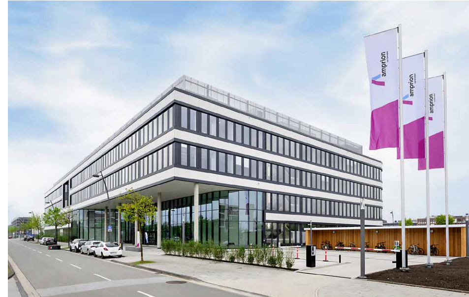
The Project Centre that opened in spring 2023 will meet 70 per cent of its energy needs with renewables.
